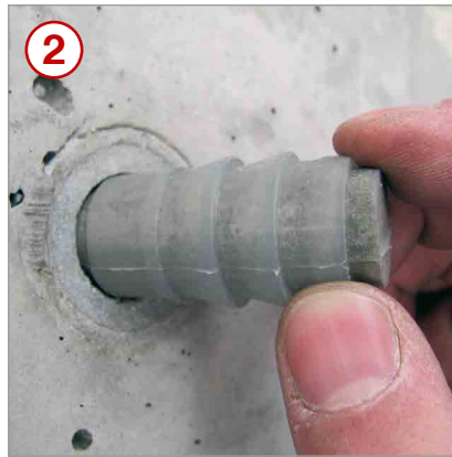
2 Insert the sealing stopper into the distance tube manually until the first sealing lip (Immersion of the sealing stopper into water makes installation easier)
