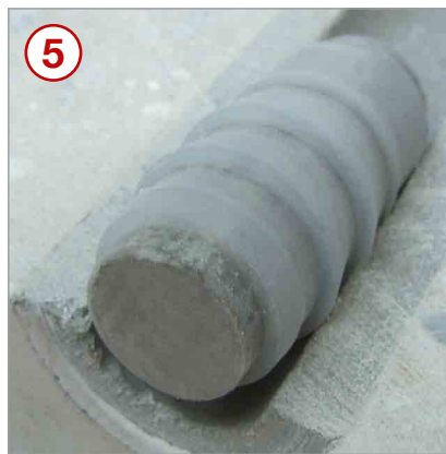
5 Cross section of the plugged distance tube
