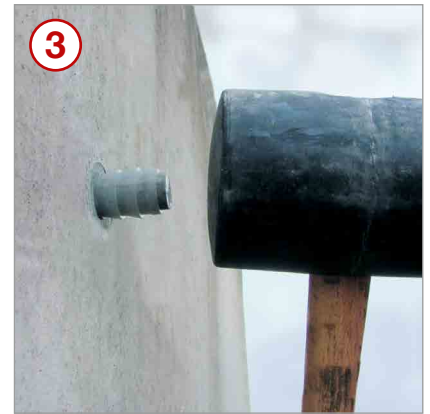
3 The stopper is driven into position using a rubber mallet
