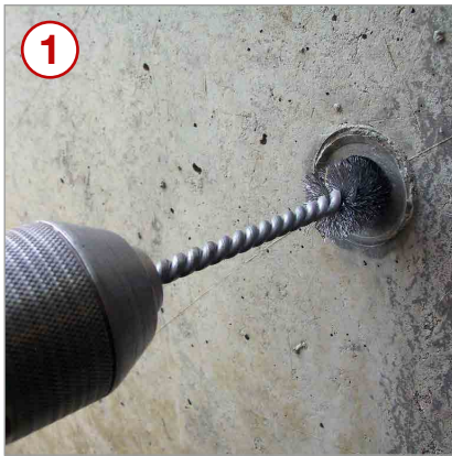
1 Cleaning of the distance tube with a cleaning brush – dust particles and concrete residues have to be removed, e.g. by blowing out
